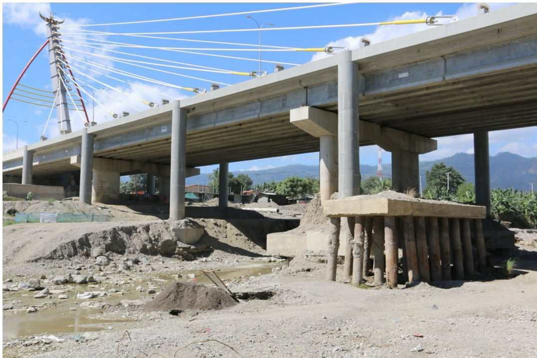
Comoro River bridge approximately where the flying fox would have been located – 14 June 2019
