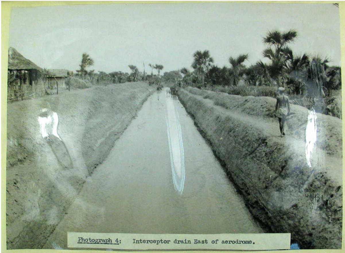
Drain east of the airfield [5]
